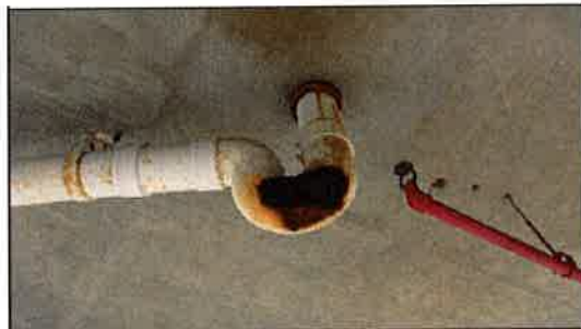
Photo 2 Deteriorated P-Trap
