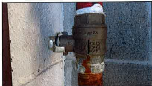
Photo 2 Deteriorated Piping
