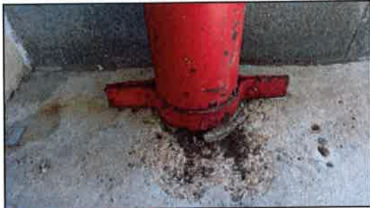
Photo 4 Deteriorated Piping
