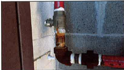
Photo 1 Deteriorated Piping
