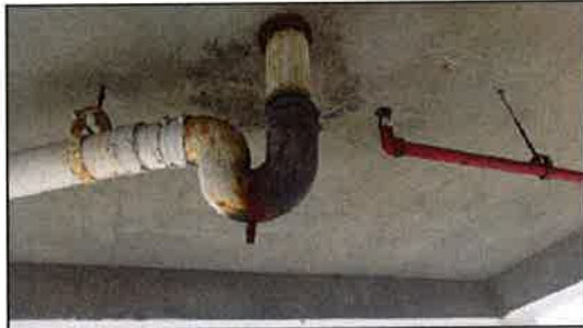
Photo 4 Deteriorated P-Trap
