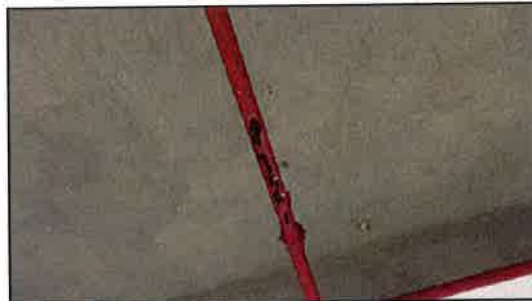
Photo 5 Deteriorated Piping
