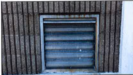
Photo 1 Remove Three Non-Active Louvers
