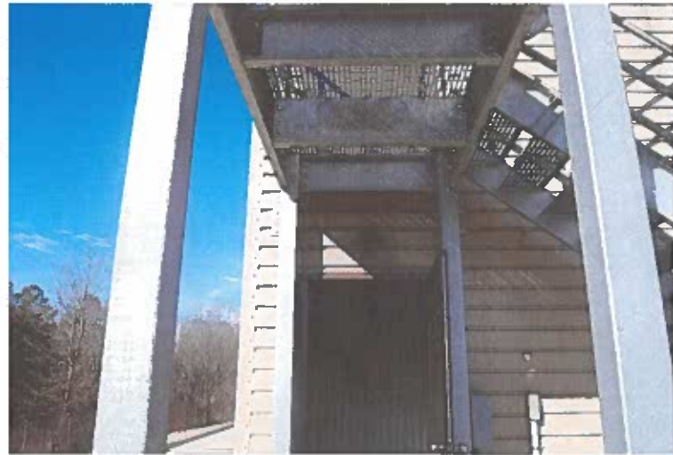
Winchester Re-Work 02-2023 022.JPG
